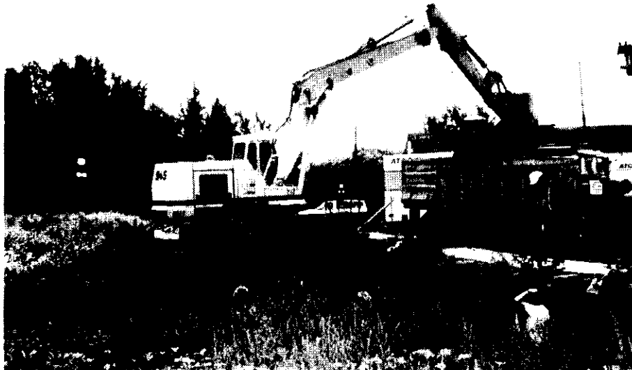
Figure 4: Re-opening the Excavation
